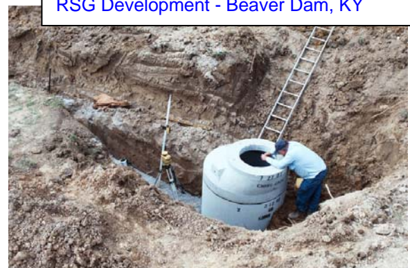
Installation of Sewer Line and Lift Station RSG Development - Beaver Dam, KY
